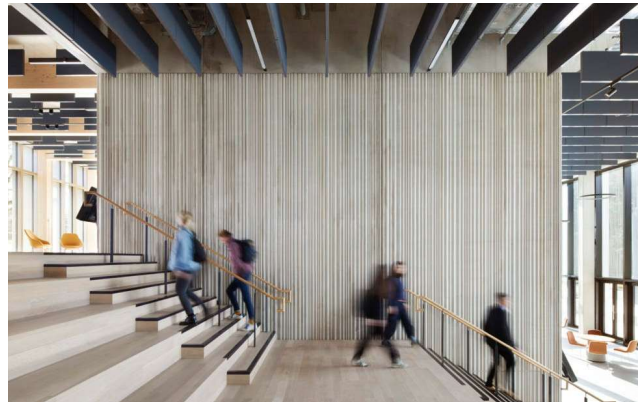
Precedent Example of Profiled Concrete Finish - IBRB University of Warwick, Hawkins Brown
