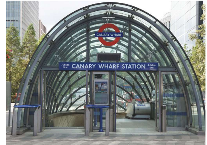
Canary Wharf Station - London, England
