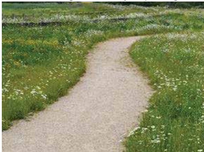
↑ Compacted gravel path
