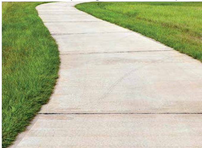
↑ Concrete footpath to road
