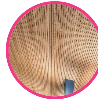
CANOPY SOFFIT Timber slatted soffit
