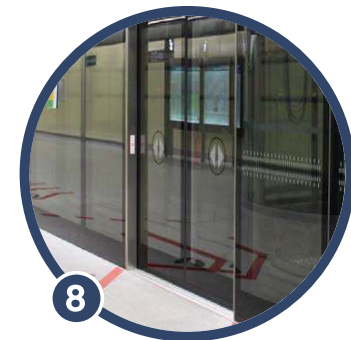
8 PLATFORM SCREEN DOORS Back painted and transparent glazing with dark metal and technical elements
