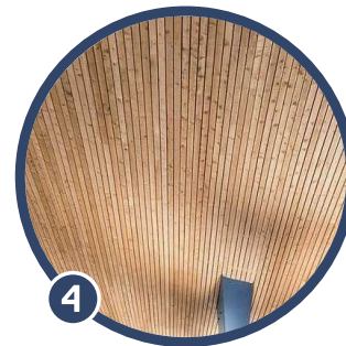
CANOPY SOFFIT Timber slatted soffit
