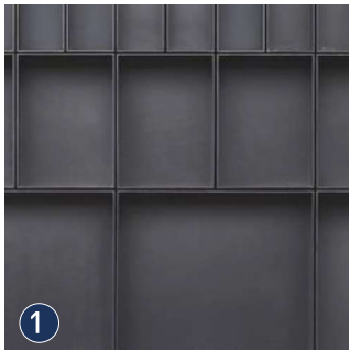
Dark metal cladding
