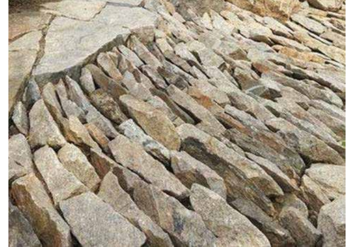
↑ Rough stone tactile surface to station pillars
