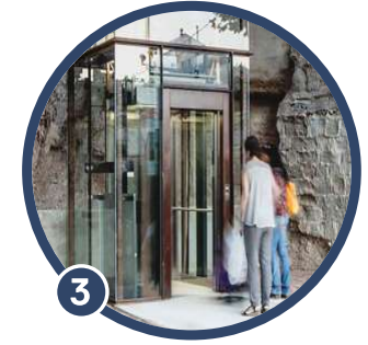
LIFTS Glazed lifts with black metal framing (frame can sit proud or be recessed subject to further design development as part of reference design stage)
