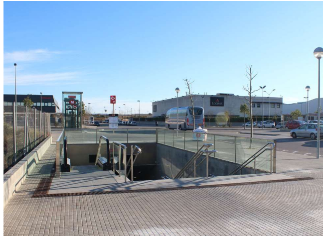
Barcelona Line 9 - Barcelona, Spain
