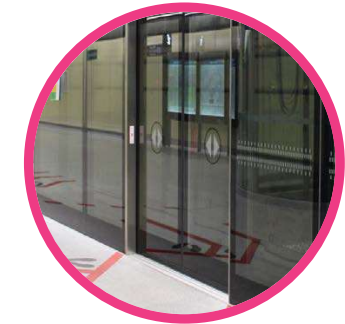
PLATFORM SCREEN DOORS Back painted and transparent glazing with dark metal and technical elements
