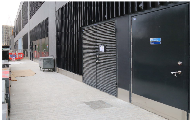
Precedent Site Photo of Dark Access and Louvred Doors - Nine Elms Station, Grimshaw
